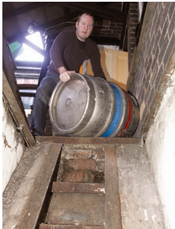
Cellar hatches present the risk of serious injury if left unguarded
